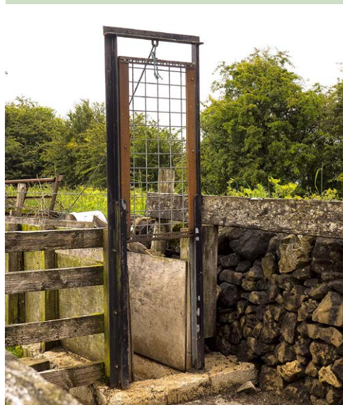
Figure 34. A vertical slide gate with rope and pulley enables the handler to operate it from behind the sheep.
