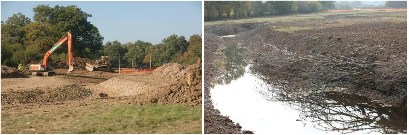
Figure 4 Re-creating natural meanders and re-profiling the river Adur channel and introduction of LWD
