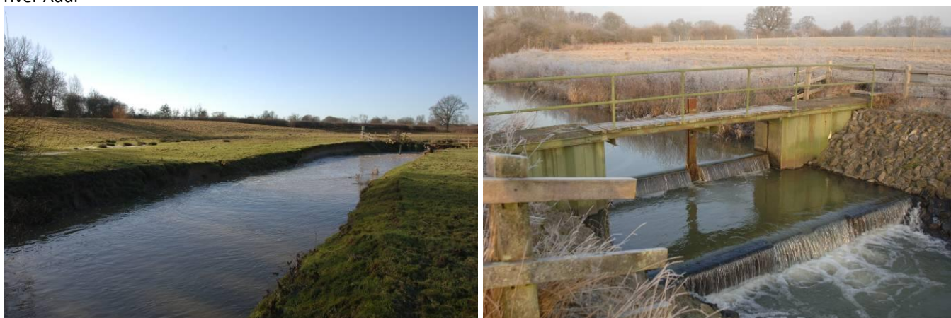
Figure 9 Canalised widened river Adur course; weir to be removed or modified to ease fish and eel movement
