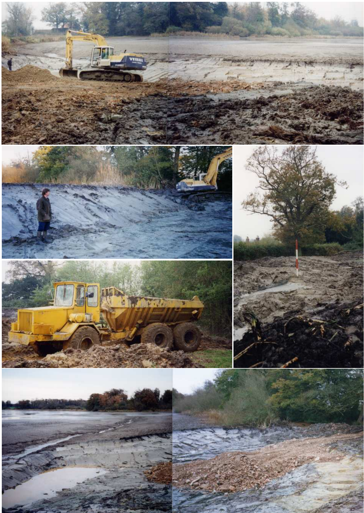
Figure 20 Photographs of dredging works in November 1996
