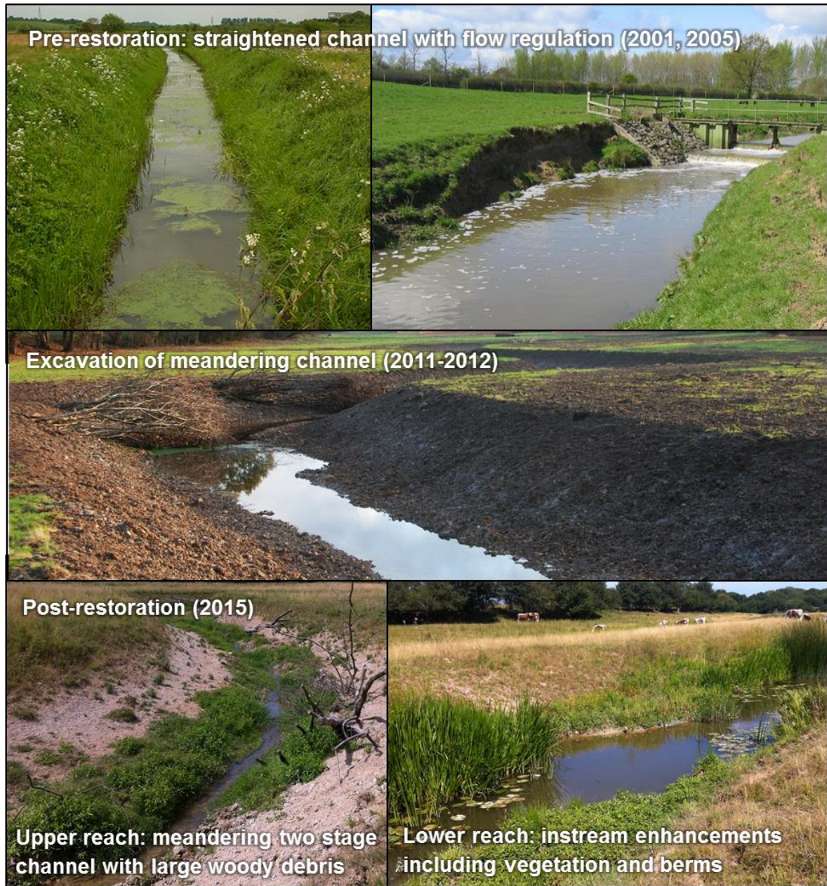
Figure 6. The River Adur at Knepp Castle Estate before, during and after restoration. Pre-restoration and restoration works are courtesy of the River Restoration Centre, post-restoration images were taken by the author.
